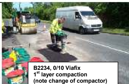
B2234, 0/10 Viafix 1 st layer placement
