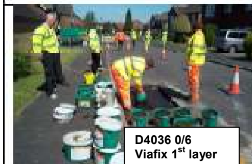
D4036, prep prior to 0/6 Viafix patch (note pavement core)
