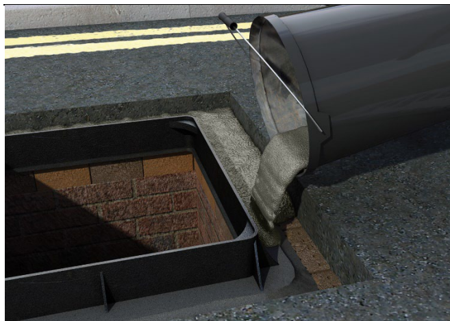
Figure 1 Backfilling using UltraCrete QC10
