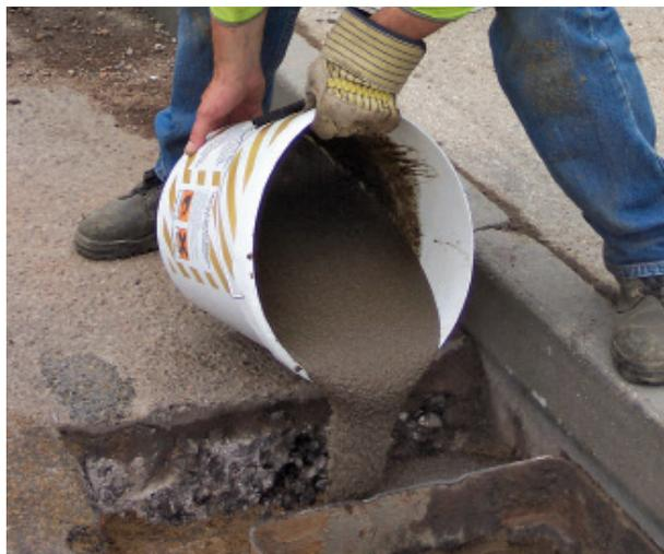
Ideal for the anchoring of bolts or bars, the bedding of lights in carriageways, backfill of manhole covers and sealing surface cracks.
