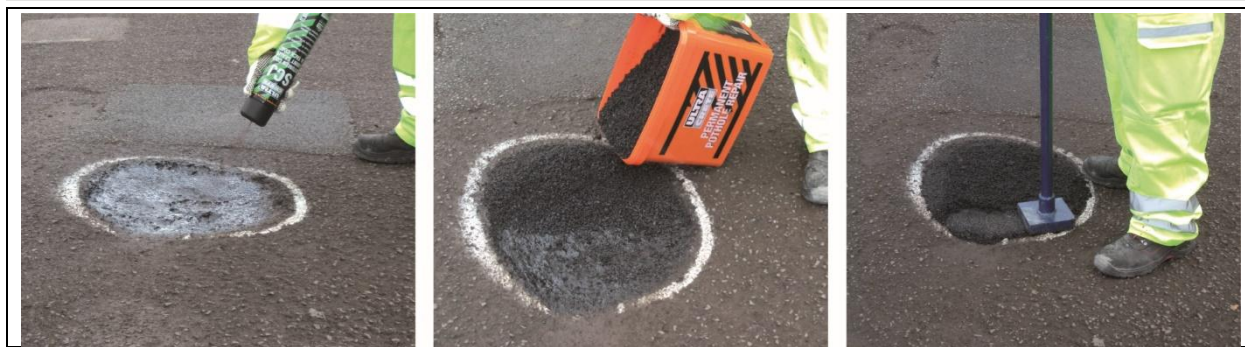
Figure 1 Reactive maintenance process
