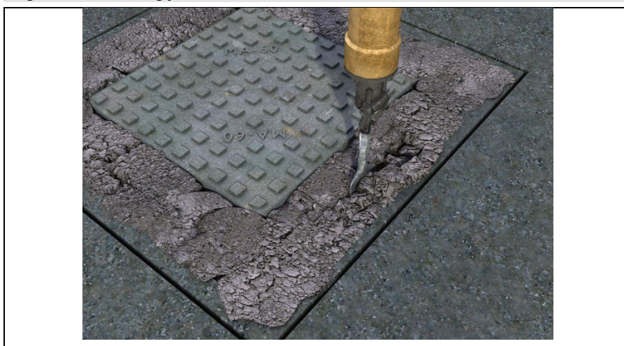
Figure 2 Excavating failed ironwork
