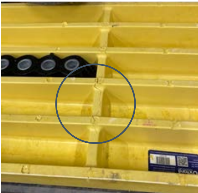
Crack along rib
