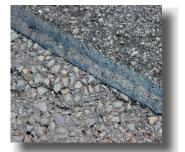
Sufficient heat has been applied once it starts to bubble, the edges of the material have settled down against the road surface and the individual pieces have fused together into one marking.
