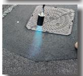
1. Clean application area thoroughly by removing all sand, dirt, chemicals and oil substances.
