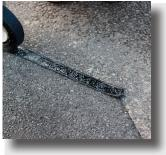
3. Place the Instaband material on the road surface with the beaded top coat facing up. Make sure it is correctly positioned at the centre of the crack.
