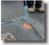
4. Heat the Instaband using a powerful gas burner (pressure min. 3 bar). Move the flame slowly but steadily 10 to 30cm over the material in a sweeping motion so that the heat is evenly distributed. It must be heated until all the material is liquid (approx 200°C).
