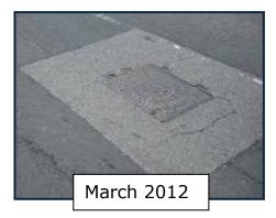
Viafix is simple and easy to use even in wet and cold conditions and permanently reinstates utility cuts and ironwork surrounds on all classes of carriageway. Viafix offers skid and rutting resistance equivalent to that of hot materials without the delays, logistical issues and wastage associated with traditional surfacing products. Viafix will massively reduce spend, risk and congestion due to defects.
