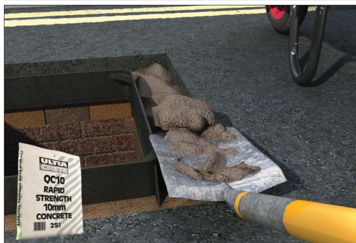
Figure 5 Backfilling using Ultracrete QC10 or Ultracrete QC10F
