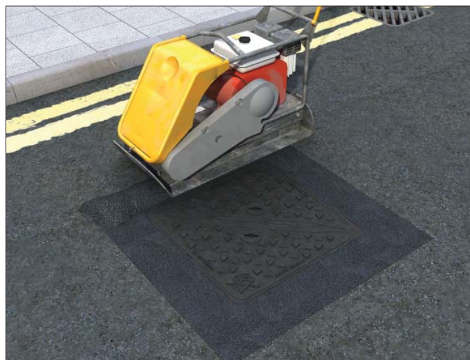
Figure 8 Final compaction of Ultracrete Instant Road Repair
