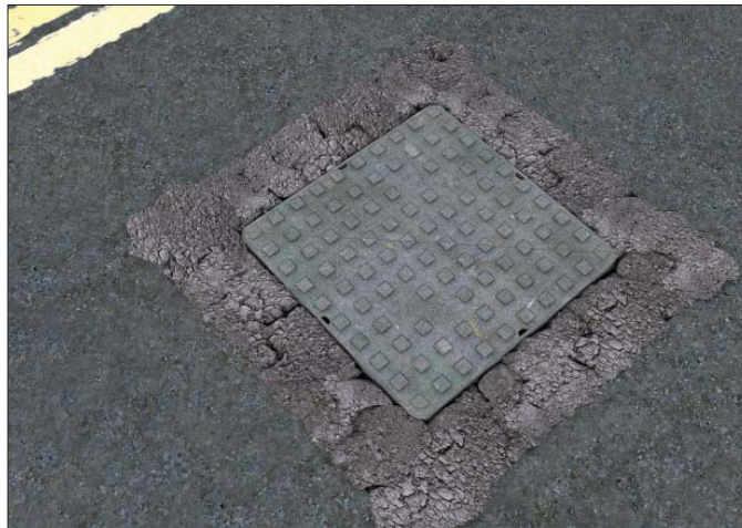
Figure 1 Failed ironwork
