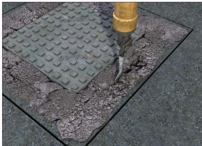
Figure 2 Excavating failed ironwork
