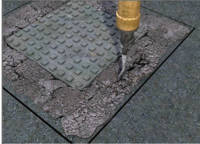
Figure 2 Excavating failed ironwork
