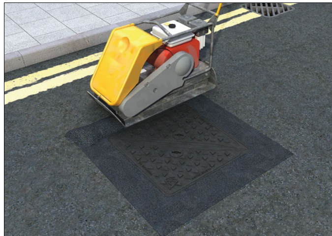
Figure 8 Final compaction of UltraCrete Instant Road Repair
