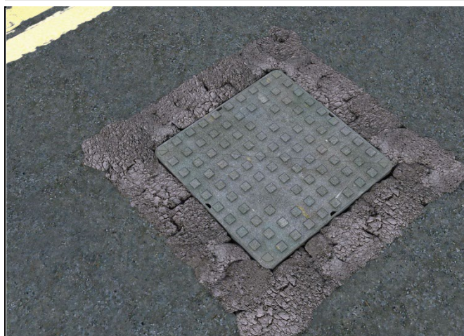
Figure 1 Failed ironwork
