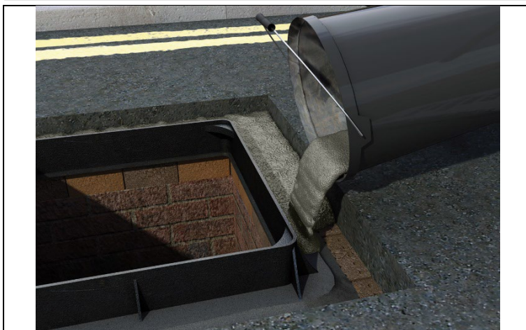
Figure 5 Backfilling using UltraCrete QC10 or UltraCrete QC10F
